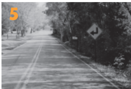
5 Right turn warning sign. Used for a left turn?
