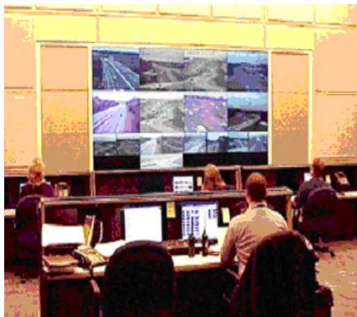
The ITS devices are monitored and operated from a transportation management center
