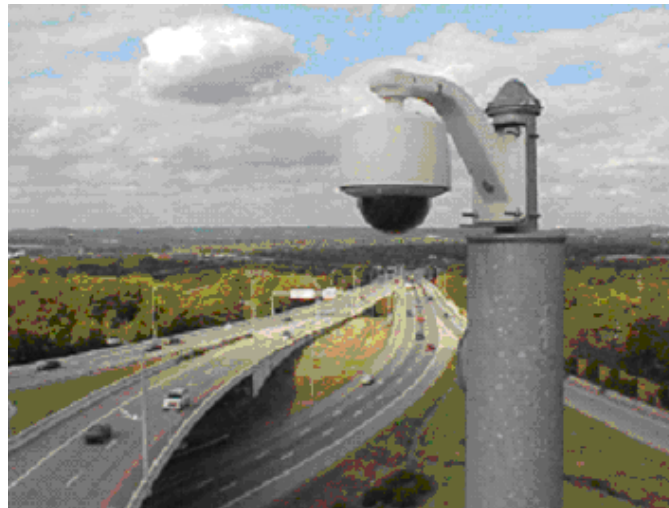
Surveillance Cameras are used to monitor traffic conditions on the freeways
