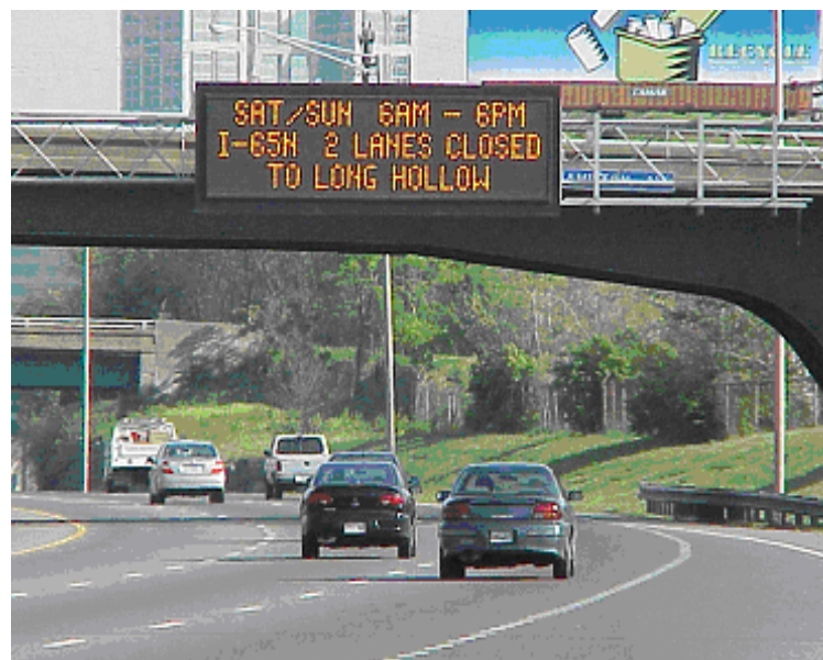
Electronic Dynamic Message Boards are used to alert drivers to any traffic problems ahead
