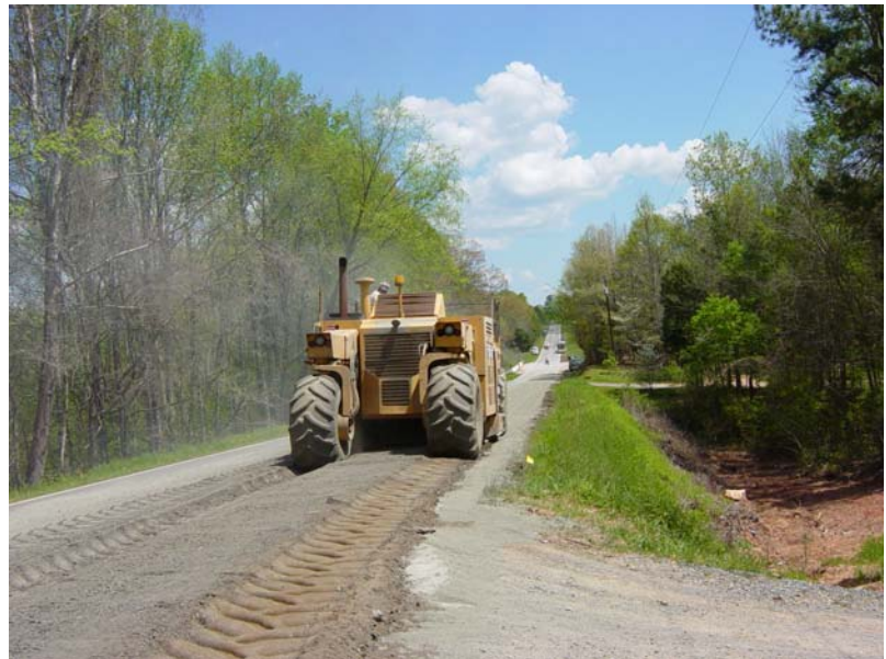
Full-depth reclamation using cement can cut costs up to 50% and will increase longevity of roads.
